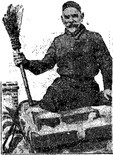
The Old-Time Chimney Sweep Has Given Way to the Giant Suction Cleaner Which Cleans Chimney and Heating Plant in One Operation.
