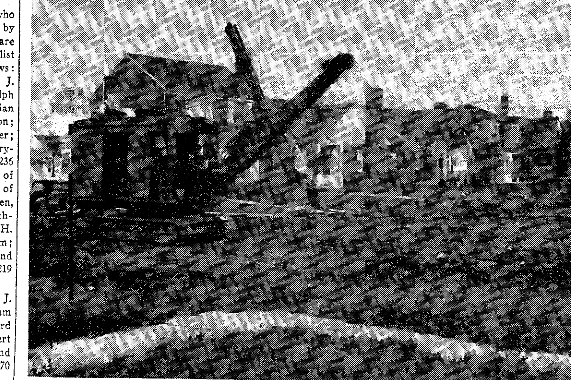
Work started last week on the paving of Beaufait road in Grosse Pointe Woods from Mack avenue to the village boundary lines.
