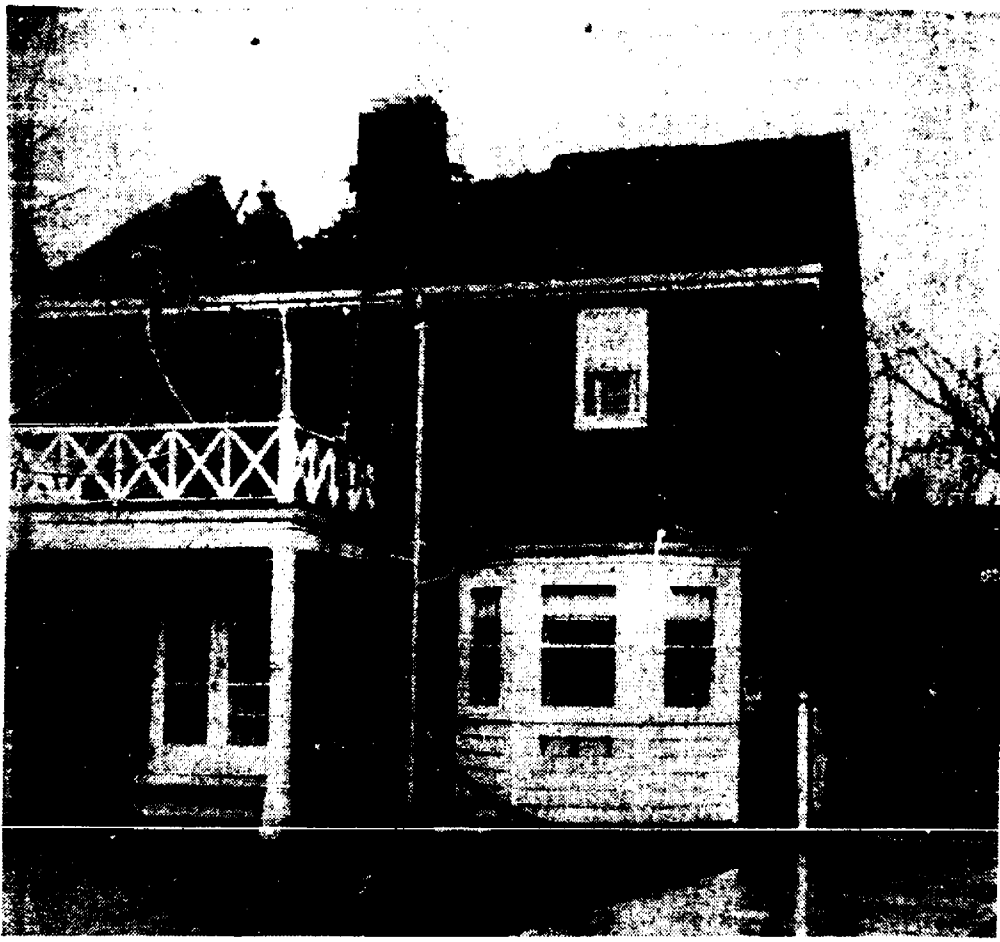
Damage estimated at $2,000 to the property and $500 to the contents of the home of the B. G. Rich's, 211 Moran, was caused by a fire of undetermined origin Monday afternoon at three o'clock. Because the entire roof was ablaze, threatening adjacent property, Grosse Pointe firemen were called to assist the Farms fire department as a precautionary measure.
