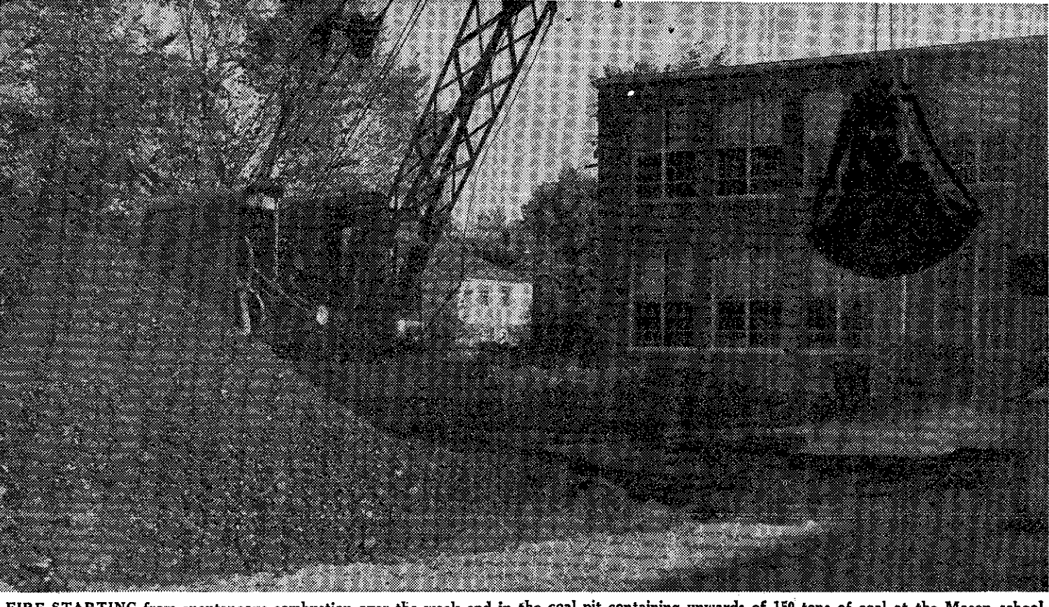
FIRE STARTING from spontaneous combustion over the week-end in the coal pit containing upwards of 150 tons of coal at the Mason school caused school authorities to dismiss school Tuesday noon until Thursday morning this week. When first discovered it was thought to be localized, but when efforts failed, a large hole was drilled through the 12-inch steel-reinforced concrete to allow the coal to be removed by the above steam shovel in three-quarter ton bites of the bucket which alone weighs 3,600 pounds. Smoke can be seen coming out of the pit and the coal taken out was subsequently spread and sprinkled with hoses. The loss is covered by insurance.
