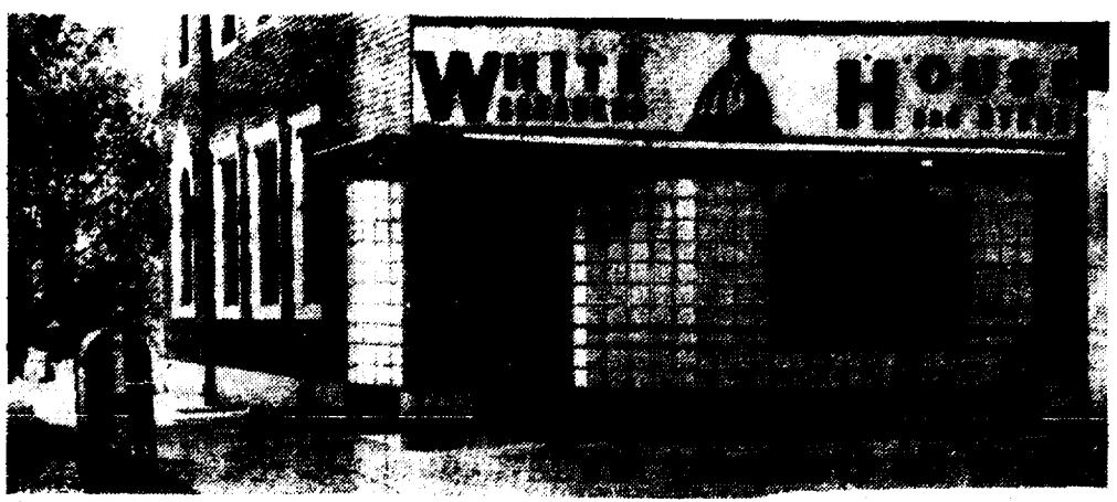
A MODERNISTIC new front greets patrons and passing traffic at White House Cleaners, popular cash and carry cleaning depot at the corner of Mack avenue and Anita, Grosse Pointe Woods.
