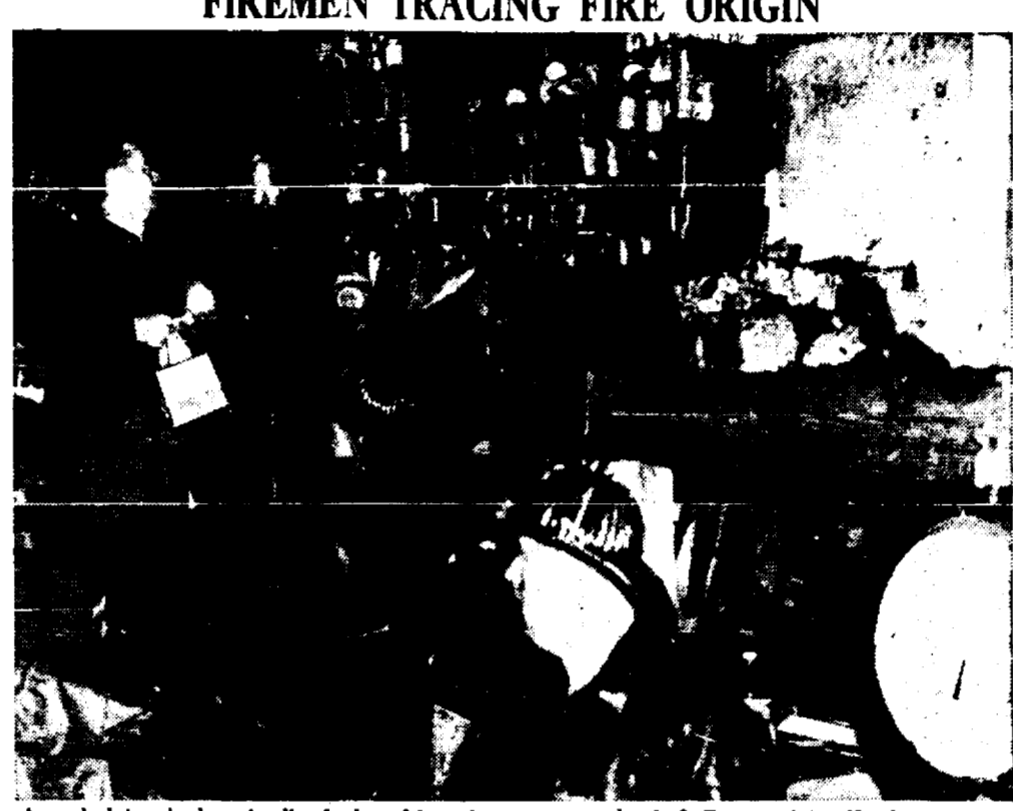
FIREMEN TRACING FIRE ORIGIN A gas leak in a broken pipe line in the refrigeration system at the A & P store, 17142 Kercheval avenue was the cause of the fire which destroyed considerable merchandise but did not damage the building. City firemen responded to an alarm at 1:30 p.m. Wednesday, Aug. 7, and soon had the blaze under control. Firemen are pictured here working to determine the cause of the fire.
