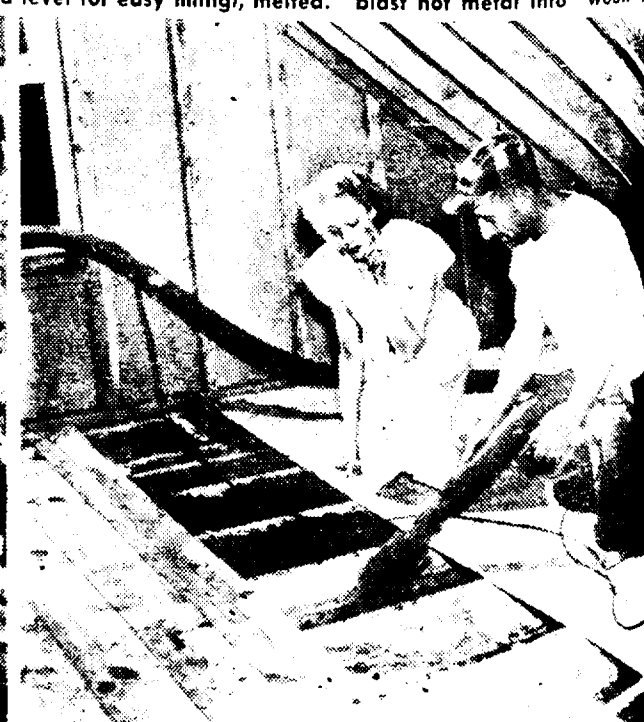
Housewife watches mineral wool in granular form being blown pneumatically into the hollow spaces in the attic floor.
