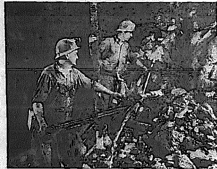
Holes are drilled for blasting charges in half-mile deep Ohio limestone mine.
