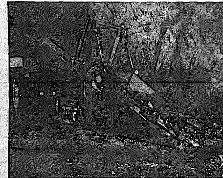
Loosened stone is whipped onto conveyor belt for speedy loading of truck.
