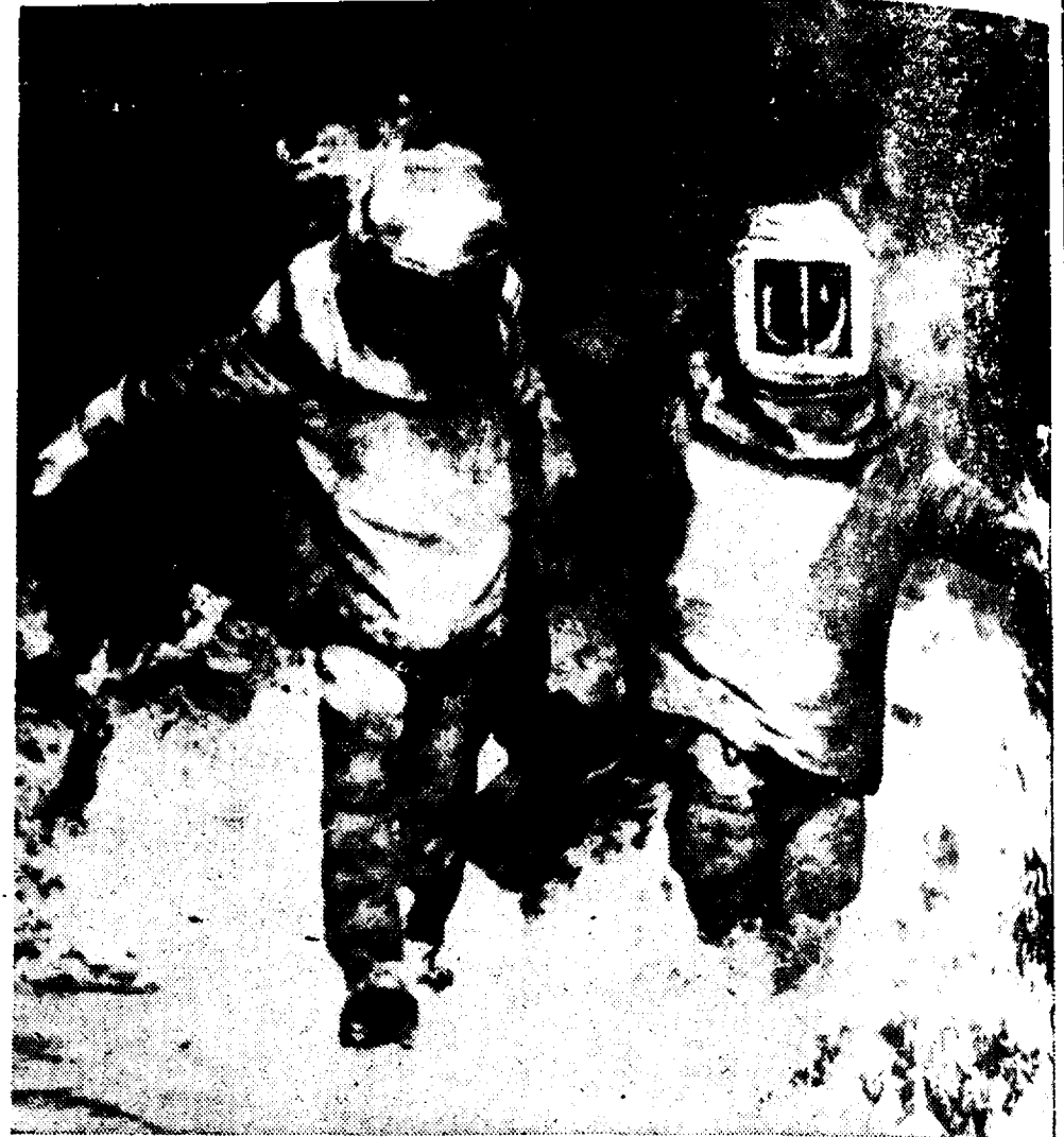
NAVY'S LATEST fire-rescue suits protect two sailors as they pull a dummy through 2,000-degree gasoline flames. New fire-fighting suit, demonstrated at the fire-fighting school of the Philadelphia Naval base, weighs only 35 pounds despite its elaborate construction.
