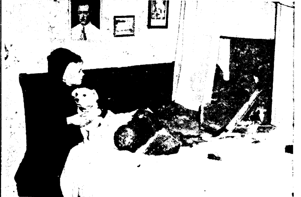
LITTLE EDWARD MANNING , 7, and his dog, Pal, look at the damage caused by a retaining wall which collapsed and crashed into a bedroom of the Manning apartment in New York City. Edward's brother, Roger, 4, was in bed ill when wall collapsed. He woke up crying. No sooner had his mother picked him up than part of wall fell on spot where he had lain.
