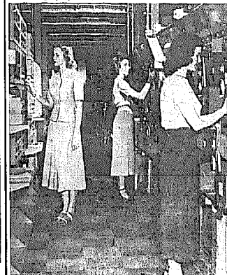
Telegrams pass through switching points in national network on perforated tape, are routed automatically to correct city.
