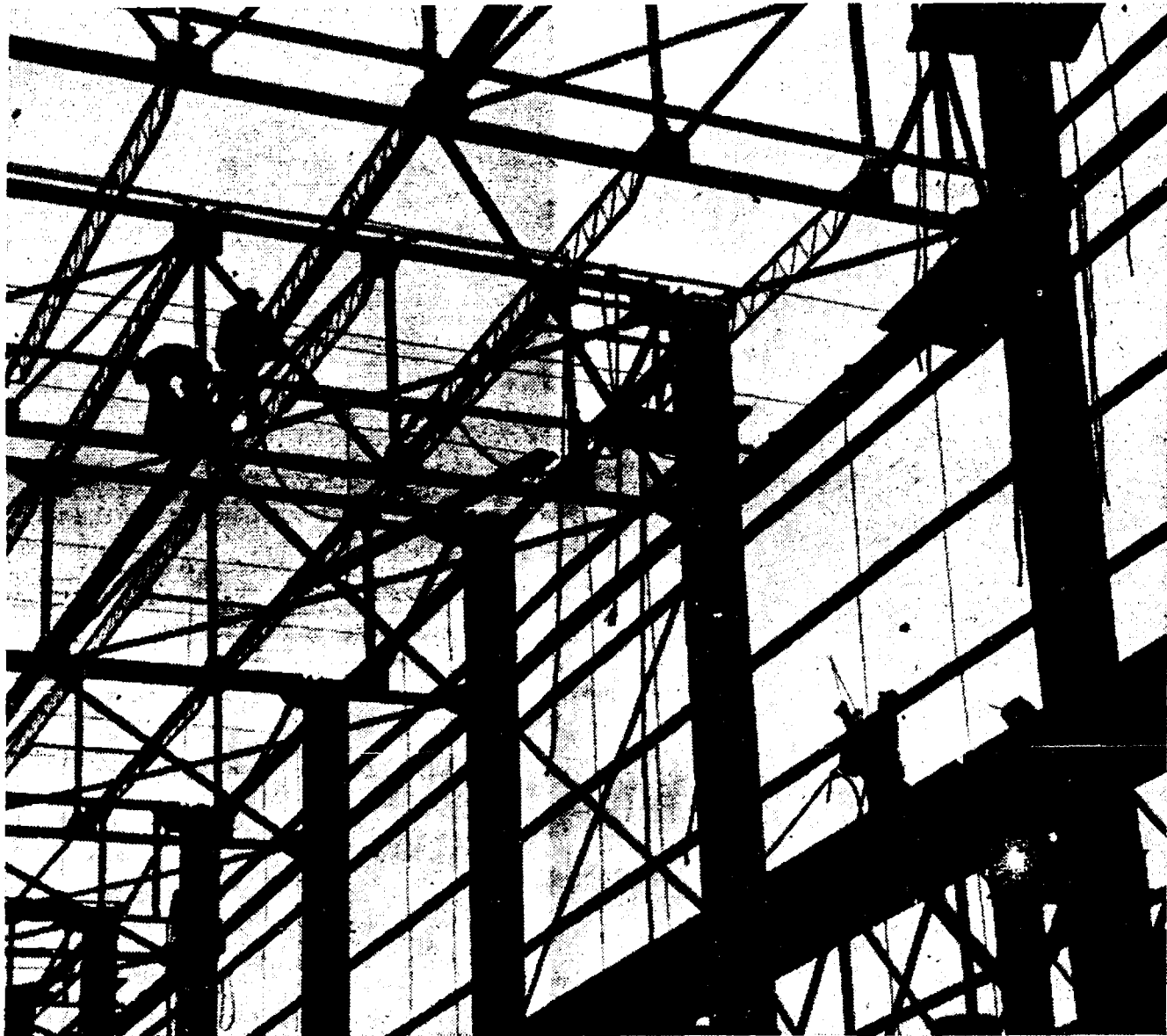
FAVORITE ACTION for sidewalk superintendents watching progress on Republic Steel's $75 million expansion program in Cleveland is the tossing and catching of white-hot rivets. The catcher is about 50 feet in the air at strip mill roll shop under construction. Approximately one million rivets will be driven home before new steel-making facilities are completed.
