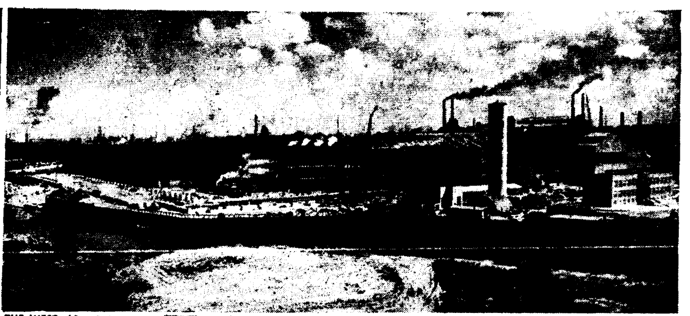
THE WEST side of the Cuyahoga river in Cleveland is calm. On the east side, noise, hustle and bustle herald construction activity as Republic Steel corporation expands operations at its strip mill.
