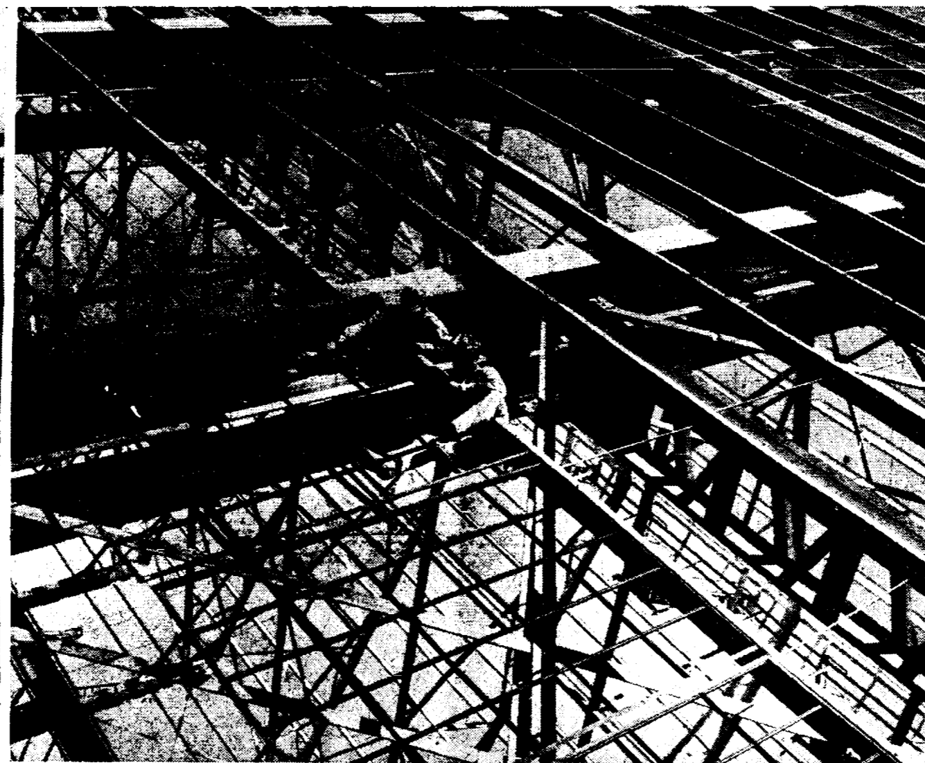
LOOKING LIKE RAG DOLLS , workmen install a window sash on a Republic Steel building in Cleveland. More than half a mile of sash is being installed in the building, part of a 75-million-dollar expansion program planned by the firm.
