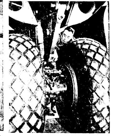
SHOCKING OCCUPATION—The landing gear of a huge bomber takes a lot of shock when the wheels touch the runway—and it's the job of Dick DeMichele to make vibration measurements in tests at General Electric Co., Schenectady, N. Y. Invaluable data is provided for design engineers on the basis of laboratory study of the gear. Although Dick's job is "shaky," he really enjoys it.
