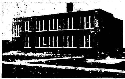
This splendid new 8-room school, The Beacon, which will open its doors for the first time for classes September 8, is situated on the west side of Beaconsfield avenue, between Woodside and Woodcrest drives. It was built with the aid of a federal grant of $58,000.00 and becomes the principal school of district No. 2, in Gratiot Township.
