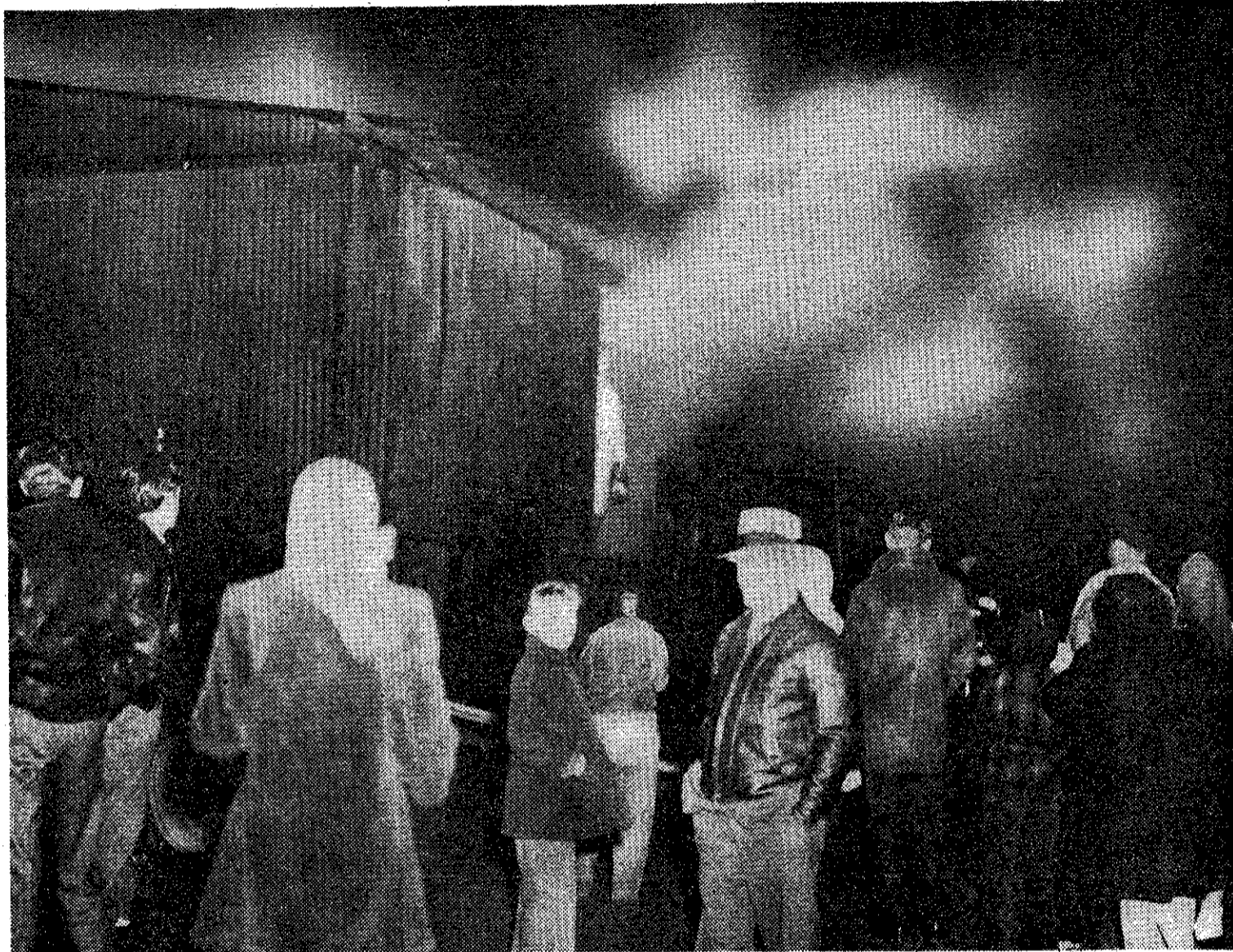
FIRE, BELIEVED CAUSED by a short circuit which developed when a truck backed into an electric wire box, broke out in the plant on Warren avenue about 7:30 Monday night. Fire fighting equipment from Detroit and the City of Grosse Pointe fought the blaze, which did damage estimated at about $3,500.
