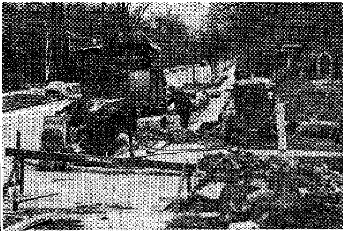
This low spot in the farms was flooded during nearly every large storm last year and in years before. To do away with this trouble, the Farms is spending a large sum to provide additional sewer facilities that will carry away the water before it floods cellars and streets. This picture was taken Monday on Ridge road, looking west toward McKinley and Fisher roads. Picture by Fred Runnells.
