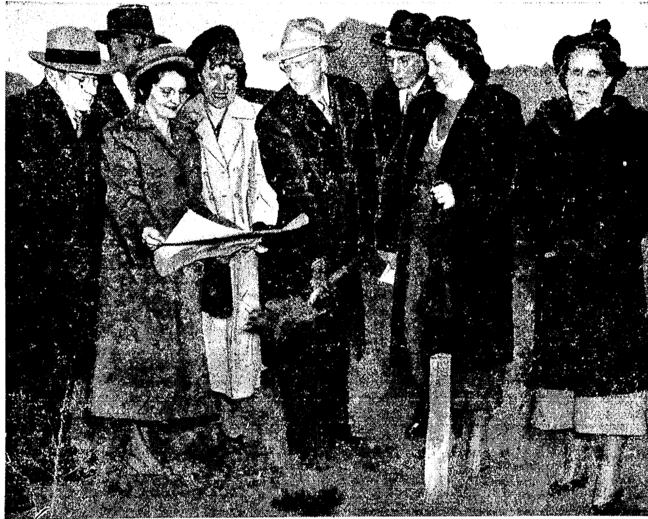
Most of the members of the small original group which started to work seven years ago on plans for a permanent building for the Grosse Pointe Congregational Church, were present Sunday afternoon when their pastor, REV. CHARLES W. SCHEID broke ground on the site of the new structure at Chalfonte and Lothrop roads in Grosse Pointe Farms. Left to right are: ALEXANDER M. MEIKLE, MR. AND MRS. J. T. HUETTE, MRS. ALTON HUNTINGTON, REVEREND SCHEID, DR. AND MRS. LYNLE R. MARTIN and MRS. MARCUS KALBFLEISCH. Missing from the original pioneers were Mrs. Wilford Lindburg and Mr. Kalbfleisch.
