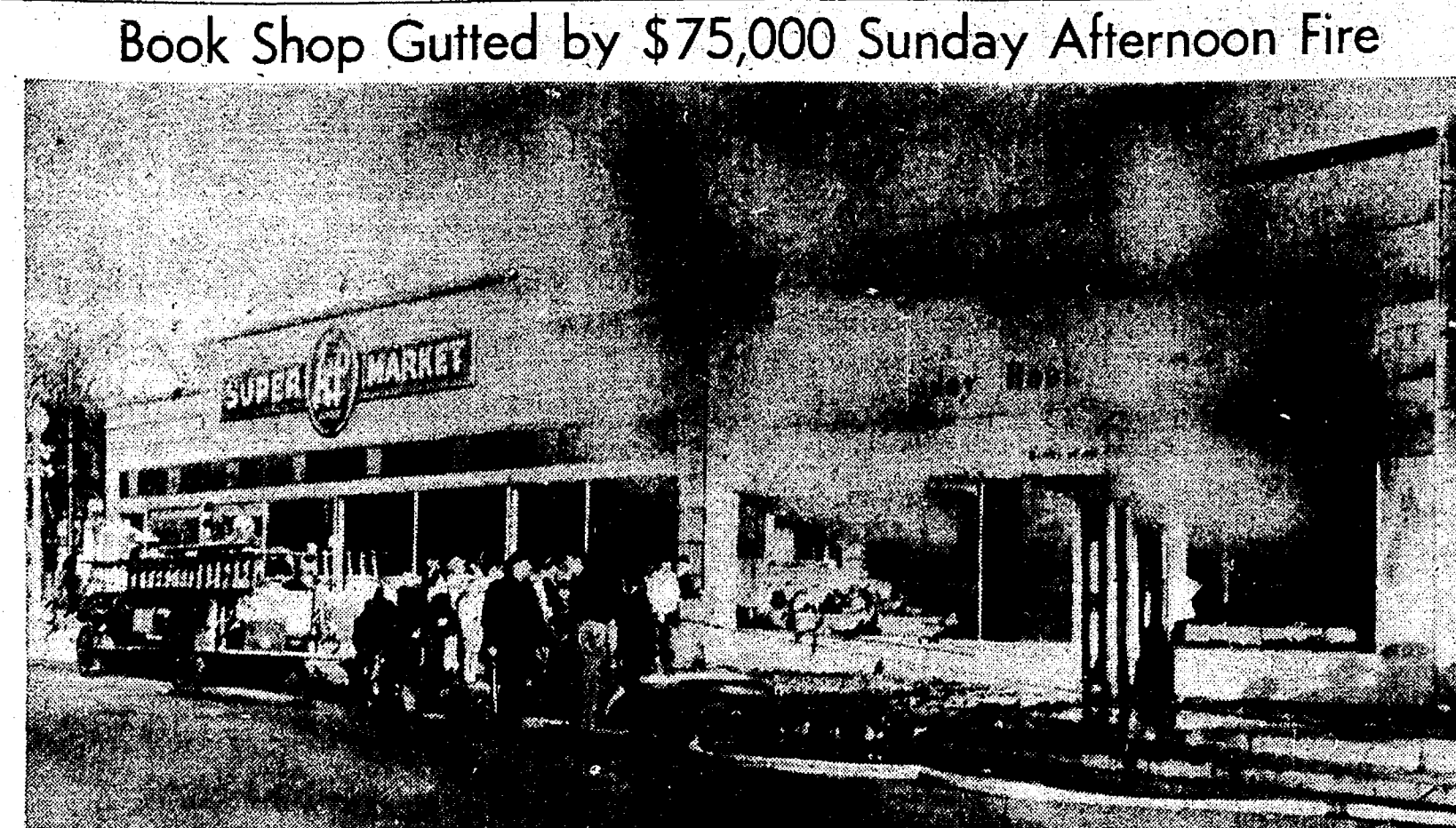
Blackened walls were all that remained of the Doubleday-Doran Book Shop on Kercheval avenue following a spectacular fire. During the height of the blaze, dense smoke from burning victrola records, books and toys lowered visibility to the near-zero point.
