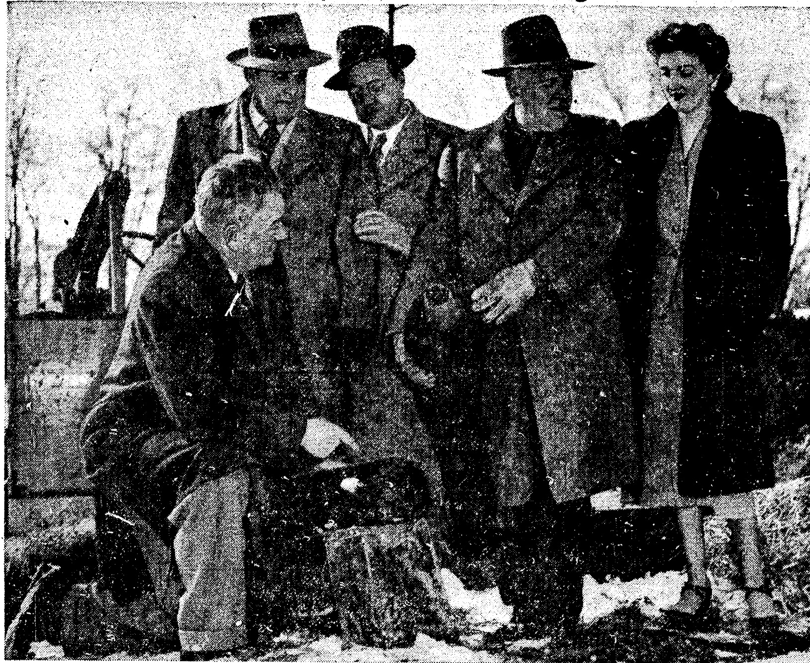
Builders digging a foundation for a new home in Harcourt road, Grosse Pointe Park, pulled up these sections of an old wooden water pipe system. NORBERT NEFF, kneeling, clerk of the City of Grosse Pointe and amateur historian of the Pointe section, says the line was laid some 80 years ago. Standing, left to right, are: EVERITT LANE, village manager of the Park; EDMUND BEAUGRAND and JACK REED, builders; and MRS. EVELYN MORRIS, owner of the property.
