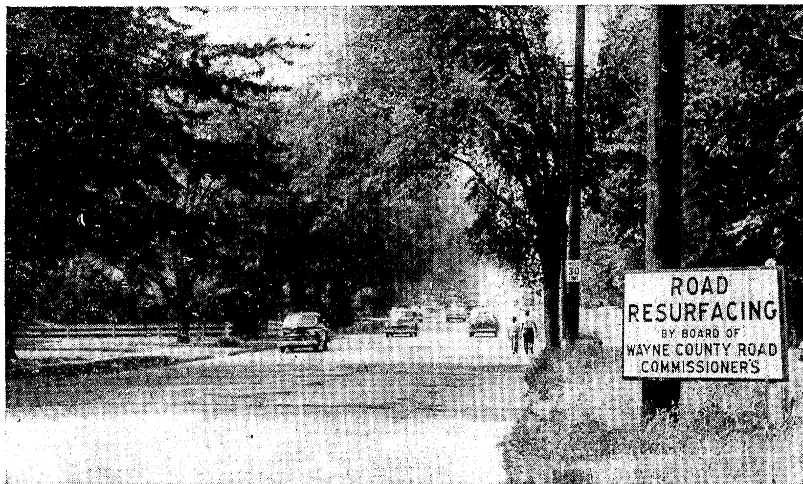
Ever since this sign was erected in Moross road some six weeks ago the question on many lips has been "Yes... But When?" The bad holes in the cement pavement have been drilled out and filled with new concrete, but that is as far as the work has progressed. The Wayne County Road Commission announced Monday that its program is so large it is having great difficulty obtaining materials and labor. It assured the NEWS that Moross road is going to get a whole new surface of two inch asphaltic concrete just as soon as possible. This work will be completed before the Jefferson avenue resurfacing project is tackled.
