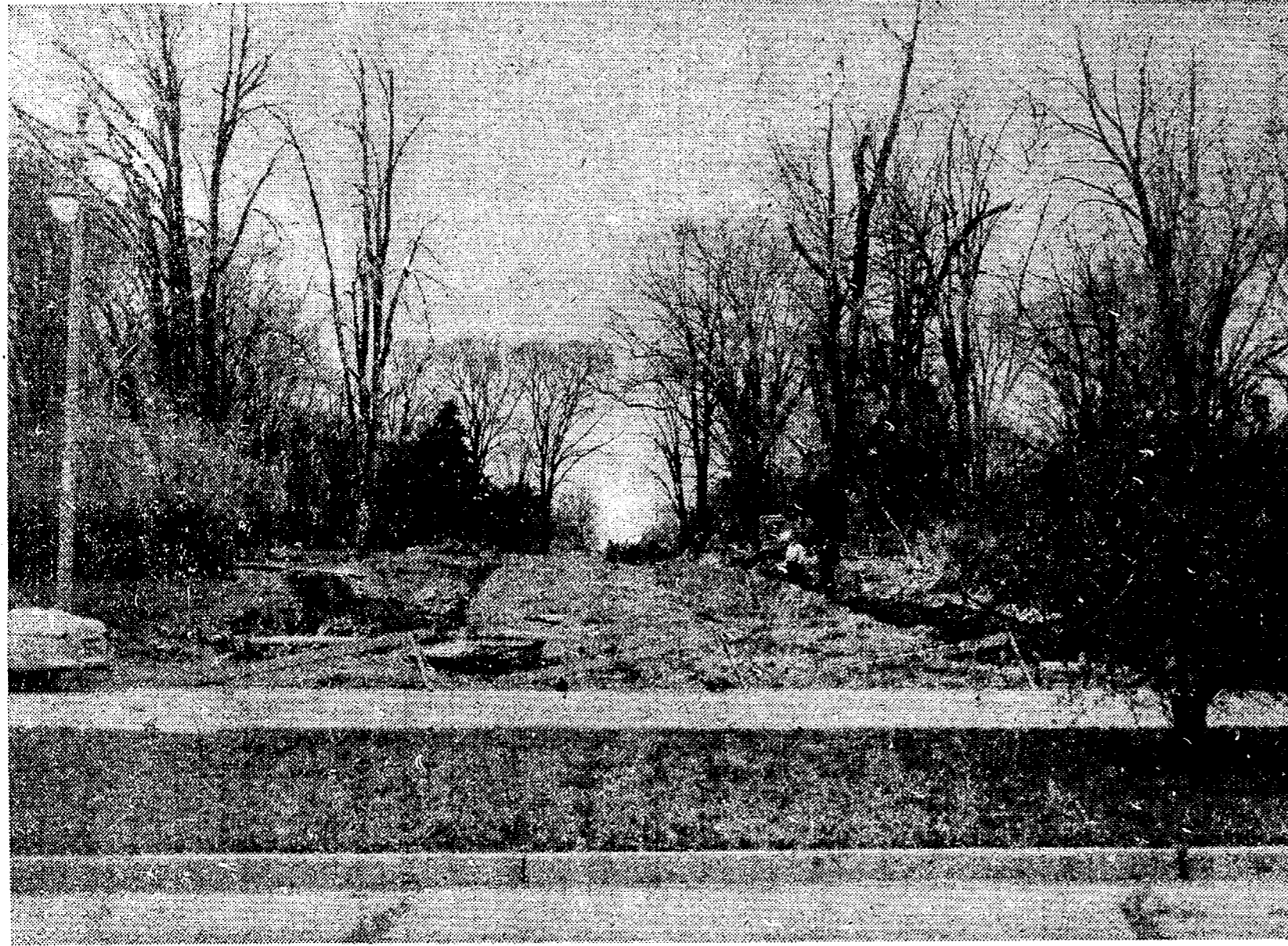
Newest subdivision along Lake Shore is that of the former Truman Newberry estate. This new road has been cut through to Grosse Pointe boulevard opposite Hall place. The newly laid concrete has been given a coating of straw to protect it from the freezing temperatures.
