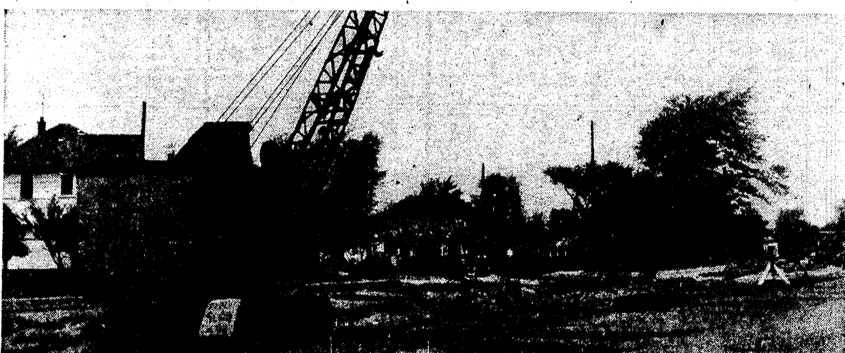
This picture, taken at Mack and Washington, shows how the old pavement, utilized as one lane of the divided highway, is being torn up to make way for the laying of a new strip of concrete. Curbs will now be installed and the roadway raised to eliminate drainage into the sidewalk area and store-fronts, which has long been a nuisance.
