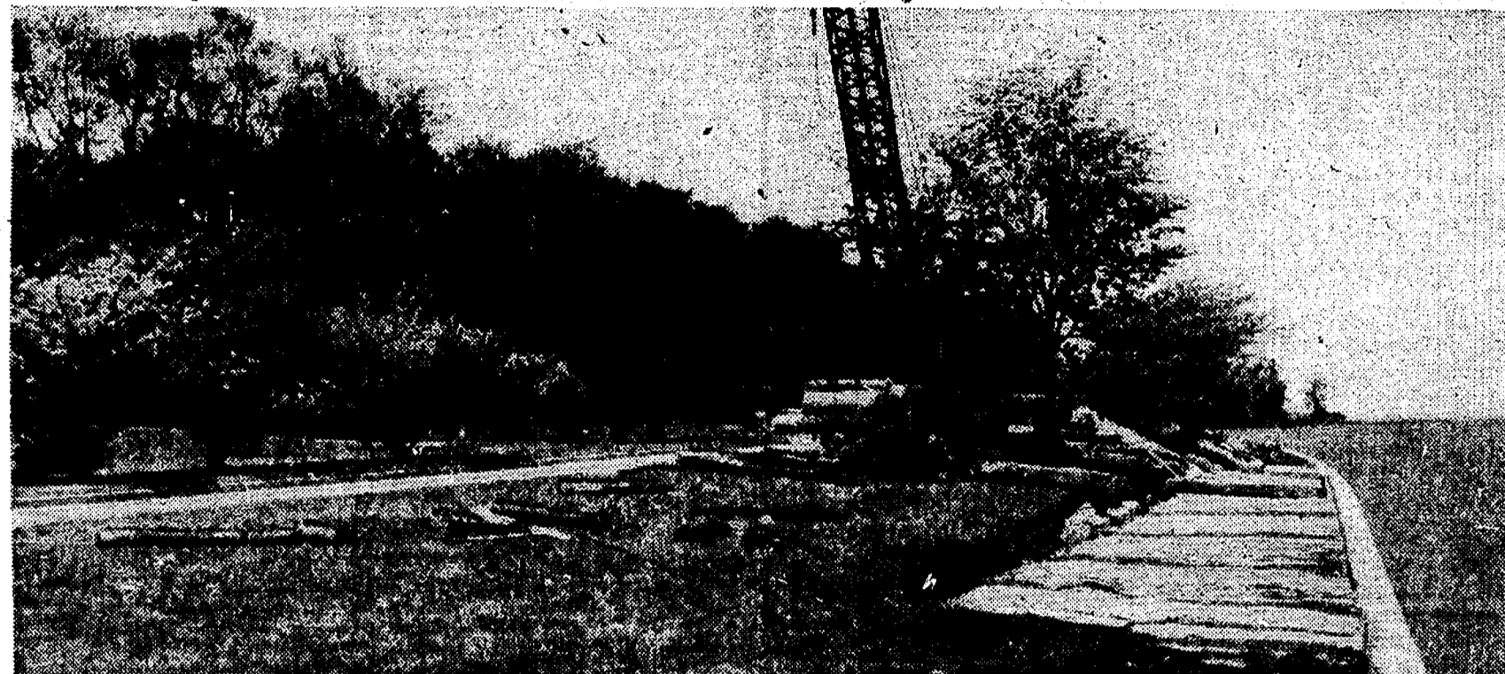
The eroded land on top of the sea wall bordering the Farms is being braced and the wall heightened by utilizing great slabs of concrete pavement being removed from Mack avenue.
