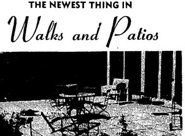
PRE-CAST CONCRETE SLABS (STEEL REINFORCED)
