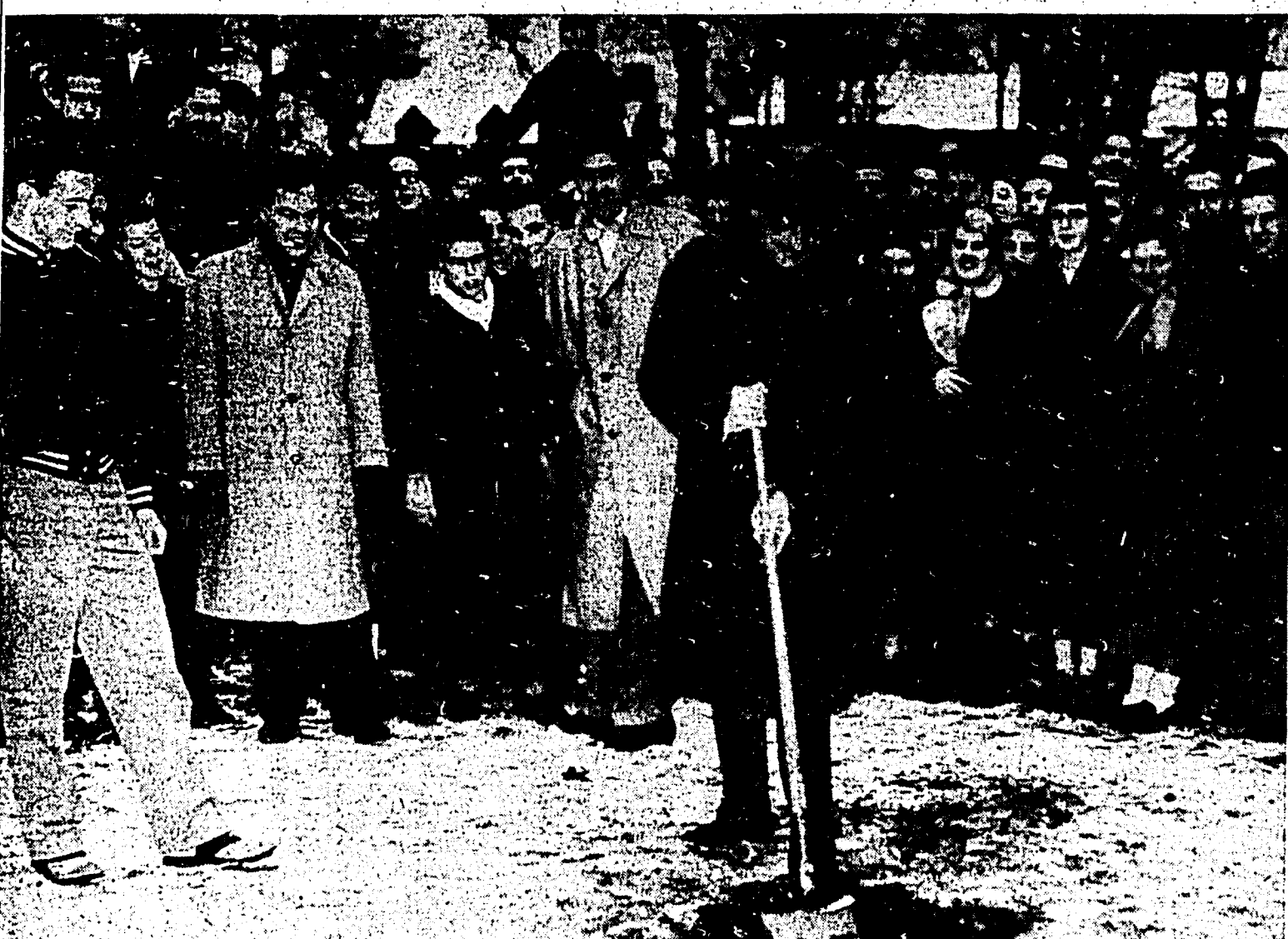
SCHOOL BOARD PRESIDENT BERT WICKING turns first shovel full of earth on site of auditorium-gymnasium, as student body and officials look on. DAVID BELFORE, left foreground, turned the second shovel full of dirt. School Board member CHET SAMPSON, in light topcoat and without hat, and SCHOOL SUPERINTENDENT DR. JAMES BUSHONG, (behind Mr. Wicking), were among the spectators.
