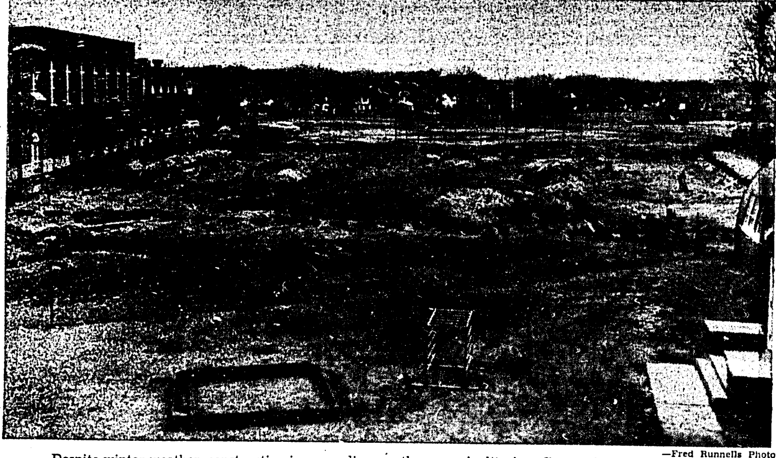
Despite winter weather, construction is proceeding on the new Auditorium-Gymnasium on the Grosse Pointe High School property. The dotted outline shows area the new structure will enclose. It is estimated it will take 320 days to complete the building, which, with fixtures and equipment, will cost close to a million dollars.
