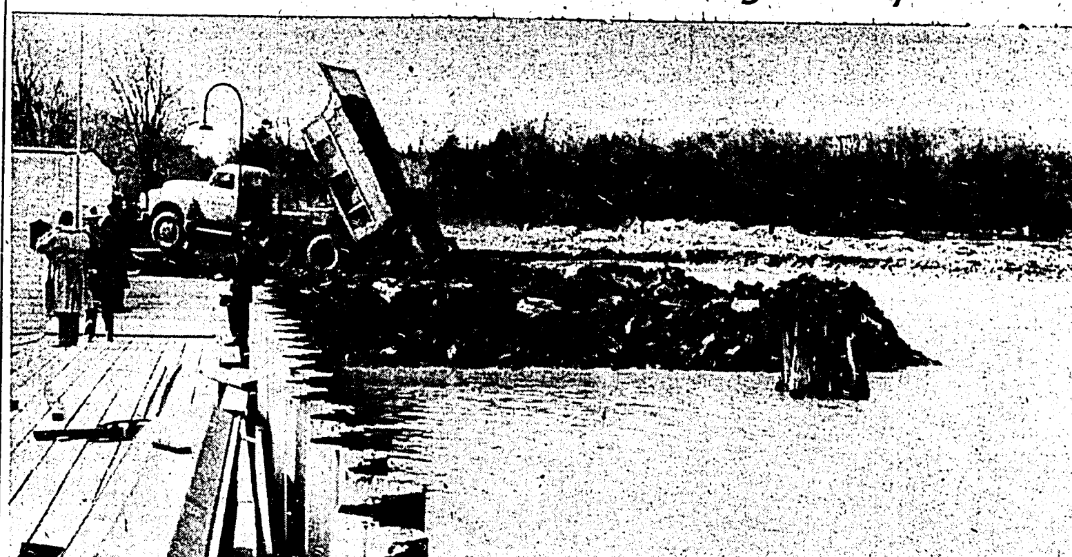
The former swimming beach at the Farms municipal park is being obliterated as hundreds of truck loads of fill dirt are being dumped to expand the picnic grounds. The big development and expansion project includes the shifting of the swimming area to the west side of the park.
