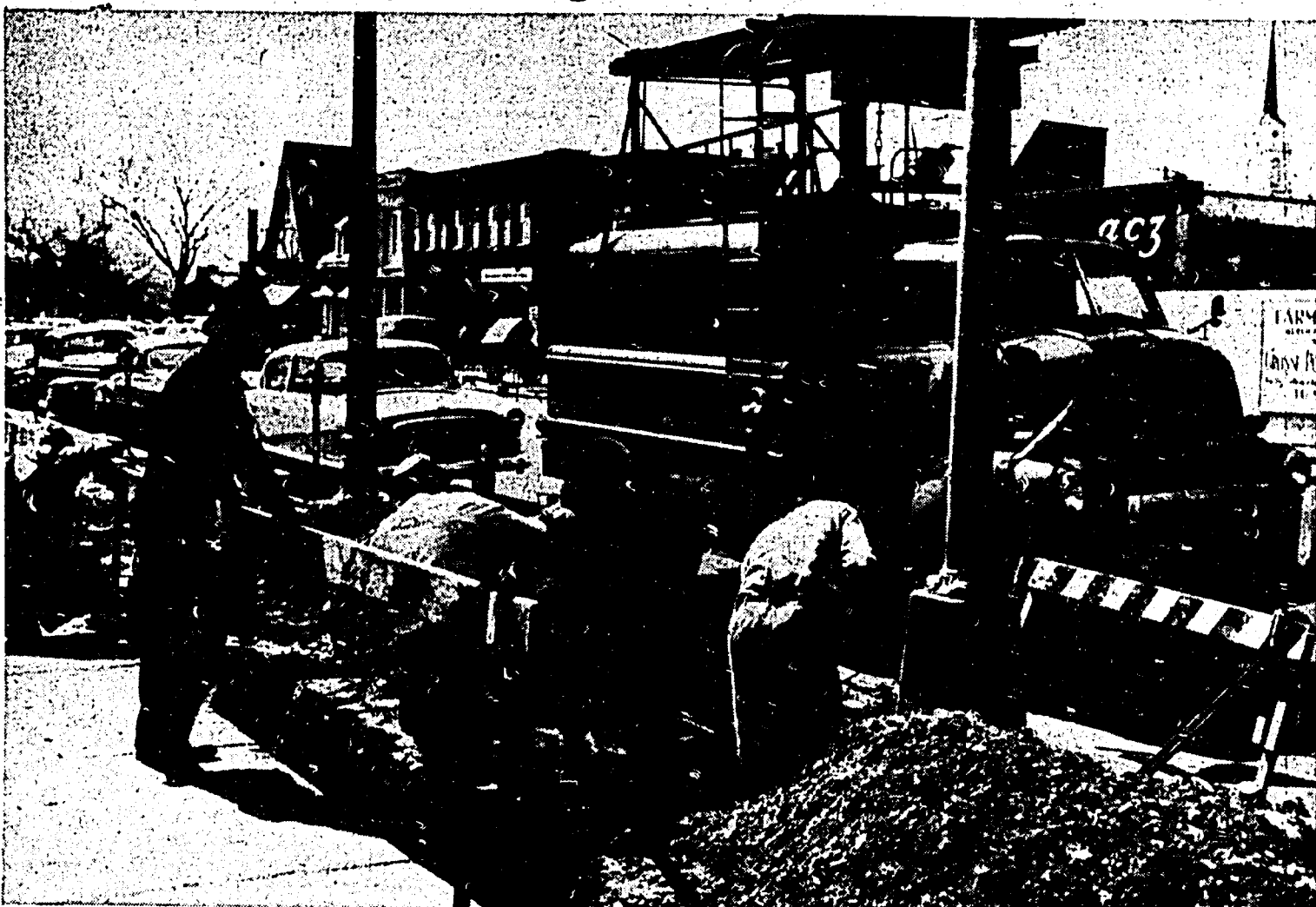
The big job of erecting new street lights all along Kercheval in the Farms from Fisher to Moross road is nearing completion. Much brighter illumination of this important thoroughfare is being achieved through the major project. The picture shows Detroit Edison workers connecting up one of the new standards across the street from the Grosse Pointe News building.
