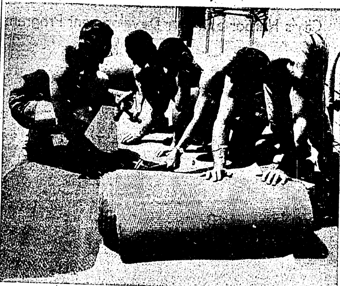
Just to prove that all is not play, as one might assume from last week's front page picture of the Farms pier lifeguards, we have here caught them in a more natural pose... working... as they wait for the pier to open. They have been kept busy doing everything from painting to laying the cocoa mats on the temporary swimming dock.
