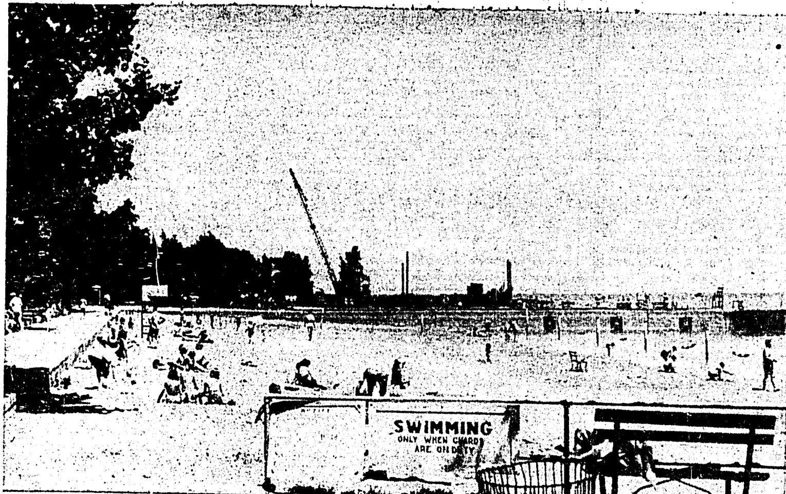
Although somewhat noisier than in past seasons, the residents of the Park can still enjoy the cool comfort of their municipal bathing beach in spite of the construction work in progress on the new boat harbor and pier. In the background, beyond and away from the swimming facilities, can be seen the pile driving rig of the Dunbar-Sullivan Co.
