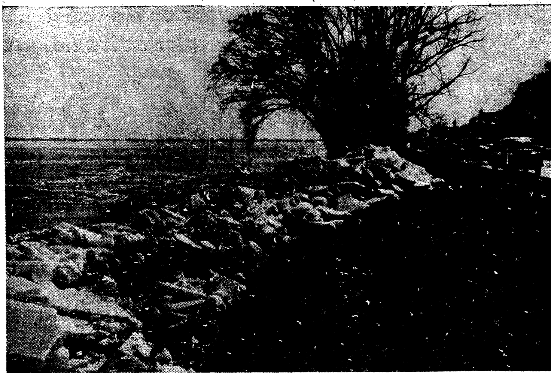
Winter is making its annual assault on the shoreline of Lake St. Clair. This picture taken at the foot of Moran road shows how huge blocks of ice have topped the sea wall, which was raised and reinforced three years ago when the rising lake caused great damage all along the Pointe shoreline.
