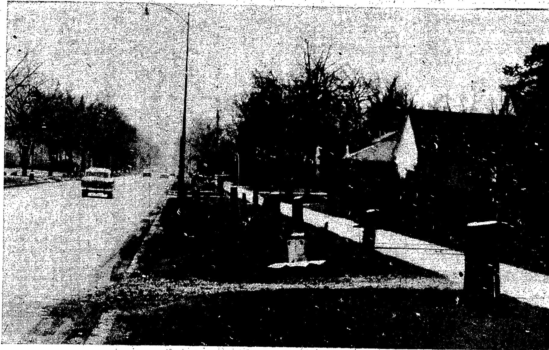
Trees along Kercheval from Moross Road to Vendome felt the woodsman's ax to make way for the new Vendome area sewer which will run from Lake Shore Road through the Joy estate and connect to sewers at Grosse Pointe boulevard, Kercheval, and Ridge Road. The sewer is being installed to eliminate flooding conditions during rain storms. The overflow during storms will empty into Lake St. Clair at the foot of Kerby Road.
