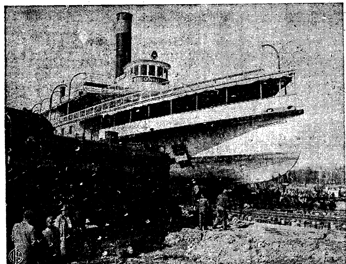
STRANGE CROSSING —This freight train had to stop, look and listen while a steamboat crossed its path on another track near Rutland, Vermont. Operations on the Rutland Railroad were halted as a special track was laid across the right of way to transport the old sidewheeler Ticonderoga overland. The operation, which looked as if someone had got his signals crossed, took a little more than an hour. The "T" is being moved nearly two miles from Lake Champlain to a museum at Shelburne, Vermont.
