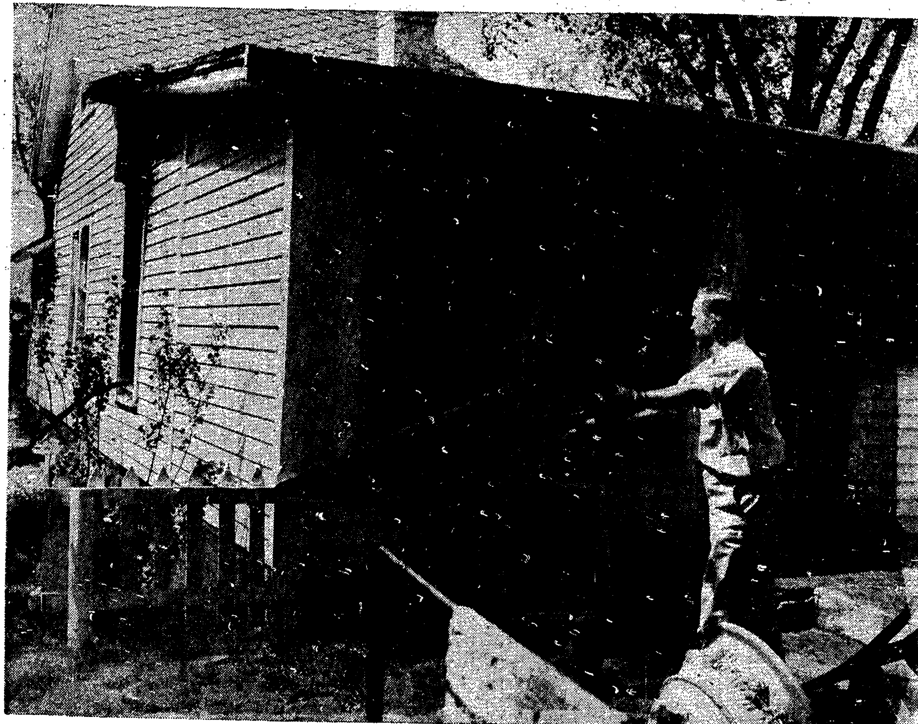
A fire in the home of Richard Debo, 200 Moross road, was extinguished by Farms firemen within 10 minutes after the Fire Department was called on Wednesday, May 4. The house, an old frame building, shown in the picture, was set ablaze by faulty wiring. Damage to the building and contents was estimated at about $6,000.
