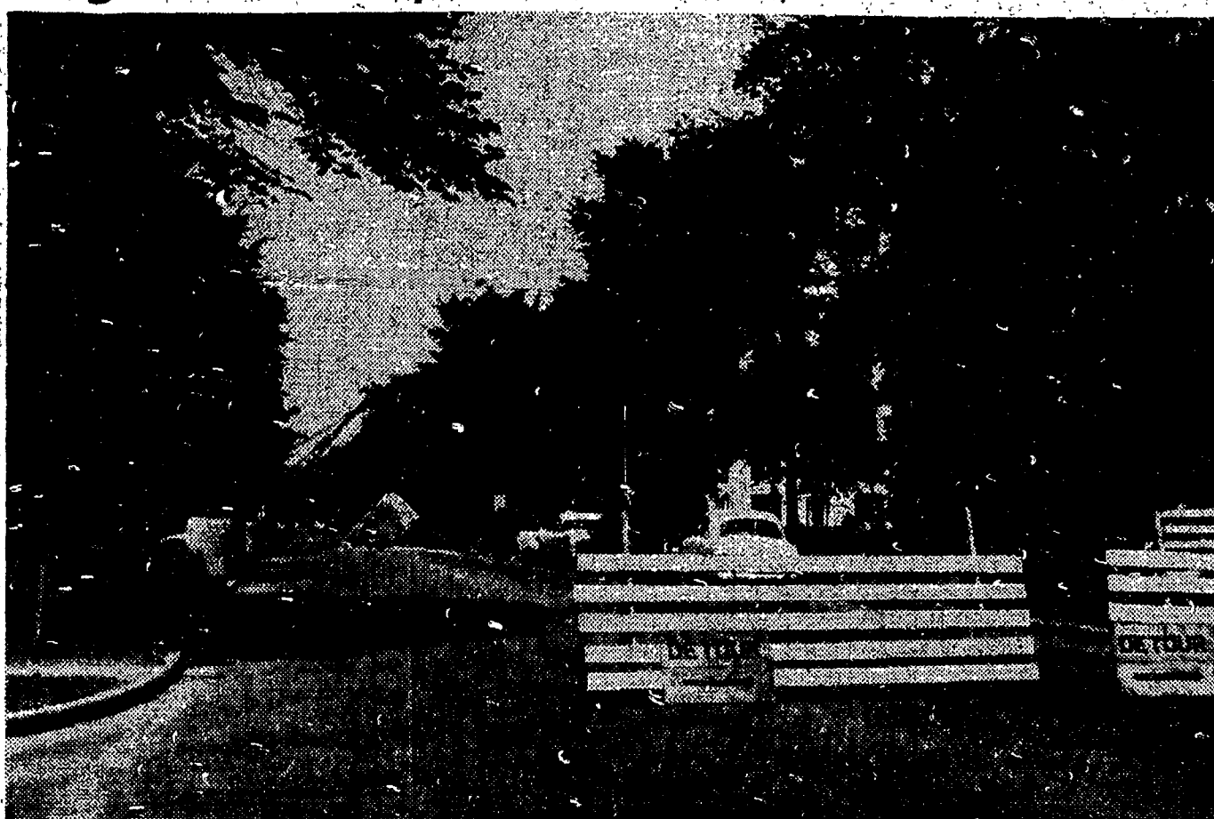
Laying of a new water main and the big new sewer main which outlets in Lake St. Clair at the foot of the estate of Mrs. Henry B. Joy, has temporarily blocked traffic on one of the city's main thoroughfares. The installation is proceeding westerly on Vendome road, from where the 21 inch main goes down Ridge road to connect with the City of Grosse Pointe's system at Fisher road. The enlarged sewer is expected to eliminate flooded basements in the Vendome area. The water main will greatly increase the supply after the filter beds are finished at the Farms pumping station.
