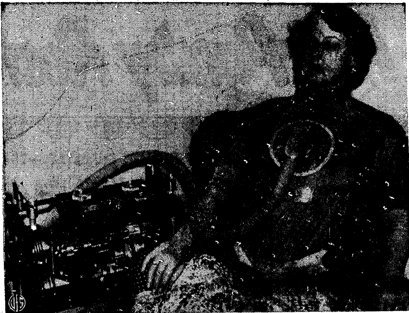
LIFE-SAVING "BLOUSE" —This portable respirator for polio victims, on display in London, is said to be the smallest in the world. Worn like a blouse, the respirator may be plugged into an electrical outlet or powered by a battery. The British-built unit is claimed to be the most advanced respirator yet developed. A special nylon fabric for the Mt. Everest expedition aided in development of the respirator.
