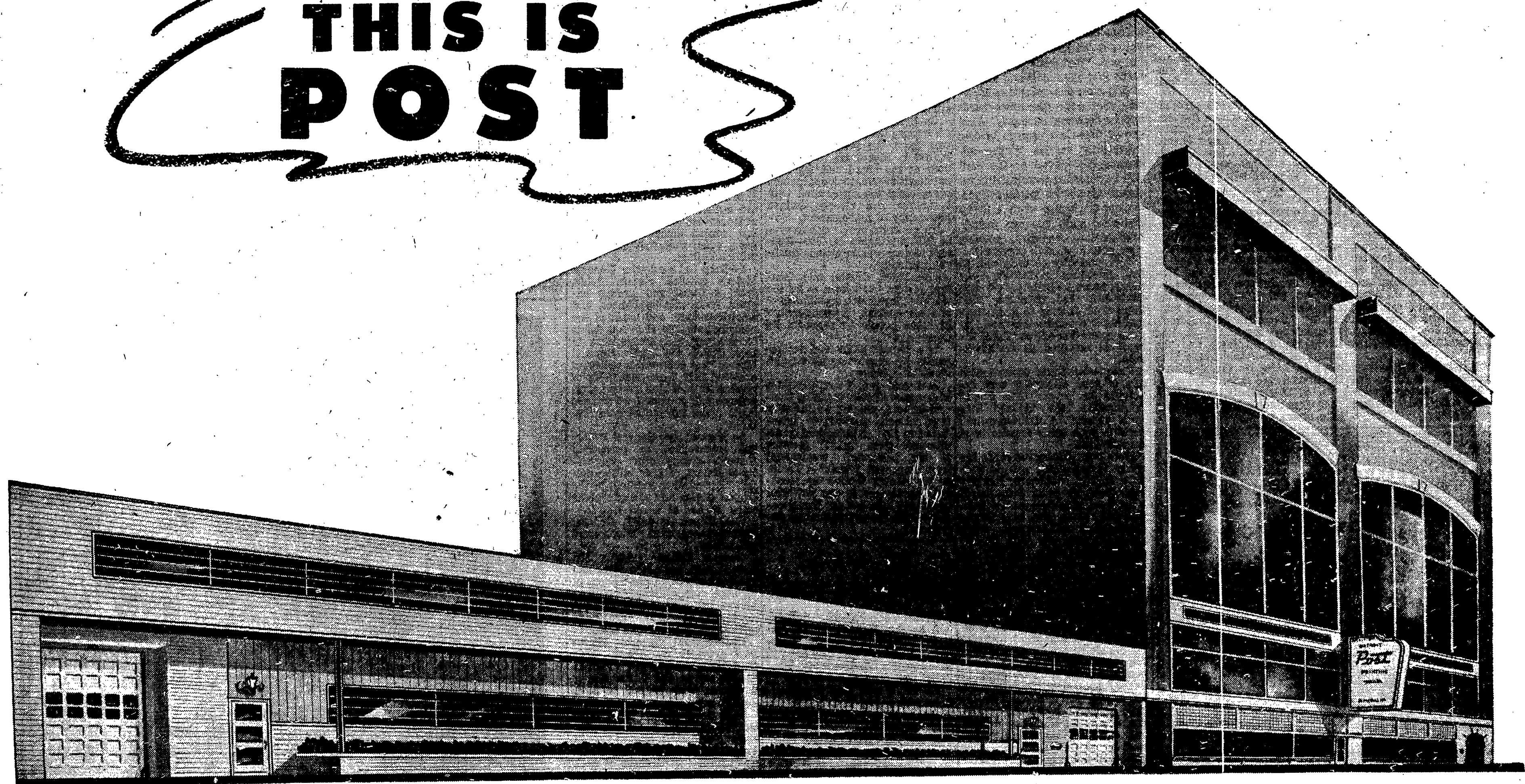
PLANT OF THE POST PRINTING CORPORATION, 1442-62 BRUSH STREET IN DOWNTOWN DETROIT
