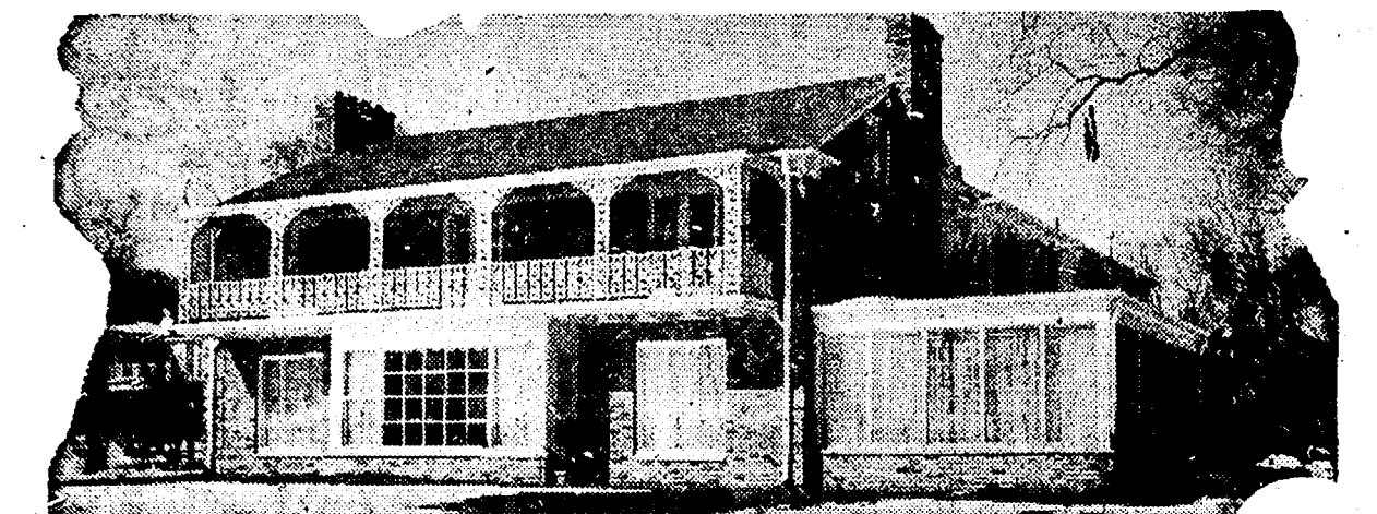
This residence at No. 10 Beacon Hill in the Farms is unique in that it is much more spacious than it appears from the street. It has a charming family room (sometimes called Florida Room) and a fully-screened upper veranda looking to Lake St. Clair and graced with New Orleans iron grill work.
