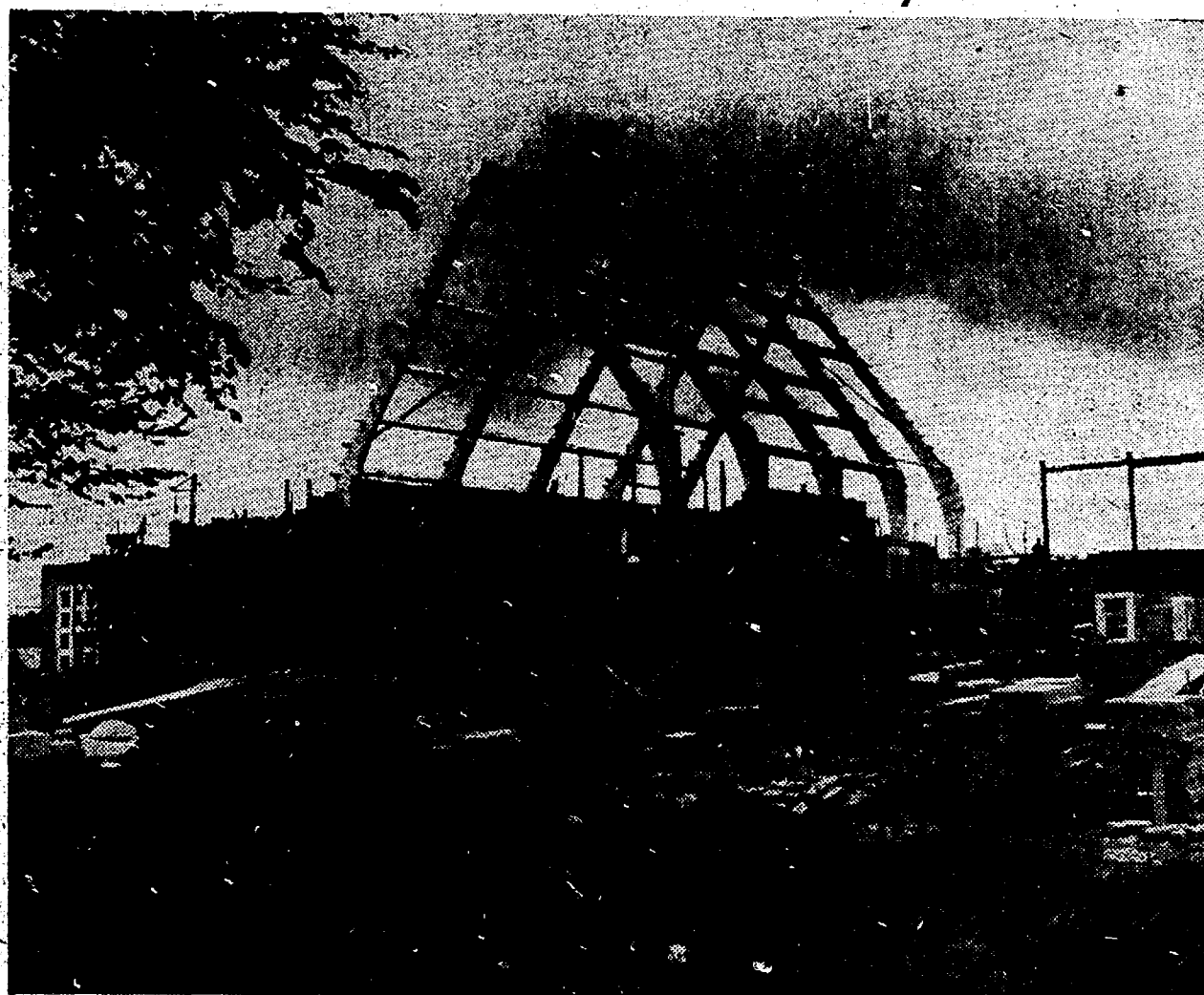
Good progress is being made on the construction of the First English Evangelical Church, being built at Vernier road and W. street in the Woods.
