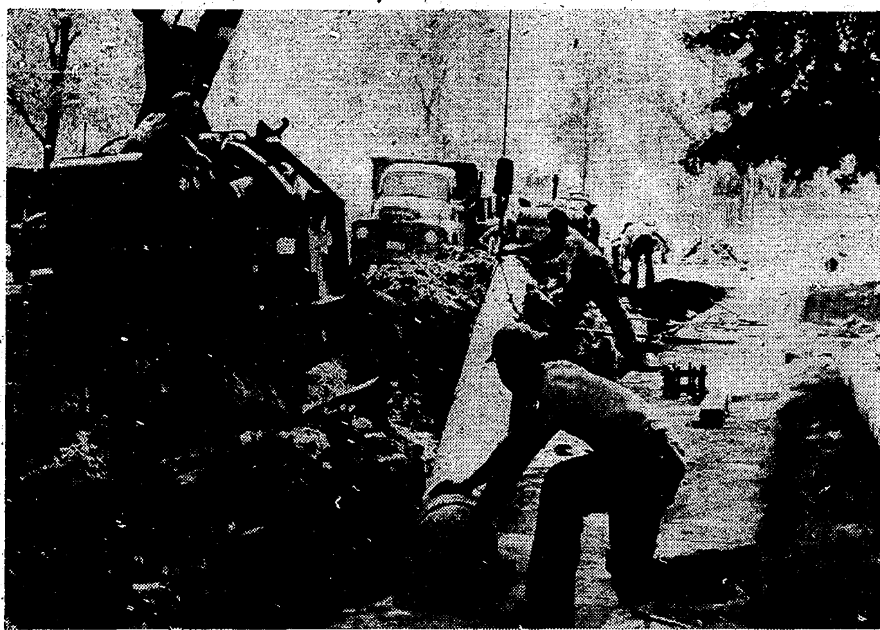
Construction men lower a section of the pipe into a trench on Vernier Road, near the Grosse Pointe Yacht Club, as work progresses on Michigan Consolidated Gas Company's new 12-inch gas main. The Company's new main is being built to satisfy the growing demands for low cost gas service in the Pointe.
