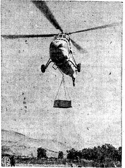
FREIGHT ELEVATOR-Lifting a load of steel and concrete, this S-58 helicopter takes the place of a dump truck, carrying men and materials across a 26-mile stretch of rugged mountain country near Santa Paula. pounds of cargo, is being used in the construction of transmission lines and towers through otherwise inaccessible areas. The experimental project is being car-
