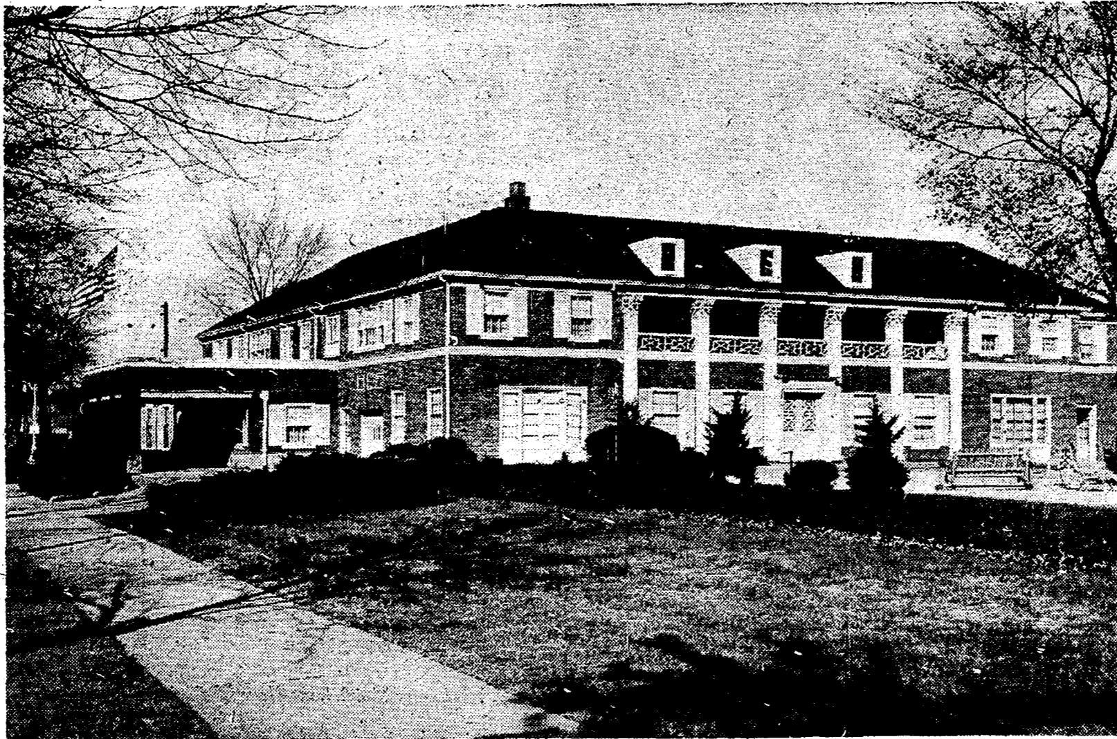
The landscaping here shows that exacting care is given far to the rear of the Verheyden property. Again it is a view from Whittier road. The Verheyden firm,
