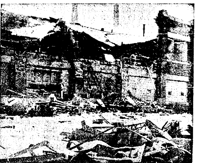
2 KILLED, 7 INJURED —Two persons were killed and seven others injured when this two-story laboratory research building at the Sinclair Oil company refinery in East Chicago, Ind., was rocked by an explosion.
