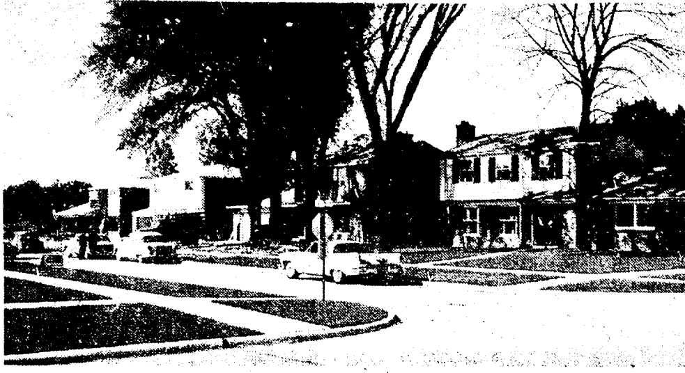
This picture of Peachtree lane shows some of the houses already completed by builder Ed Schultz, and others still under construction.
