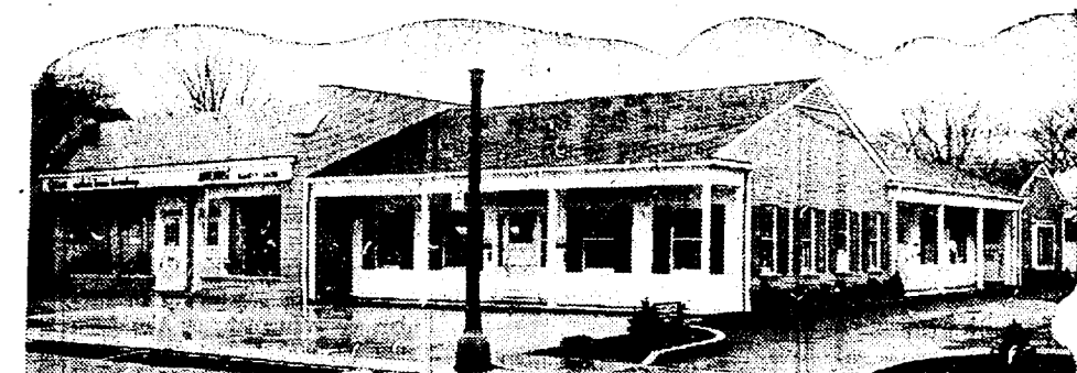
FISHER ROAD at ST. PAUL Architect, John L. Pottle
