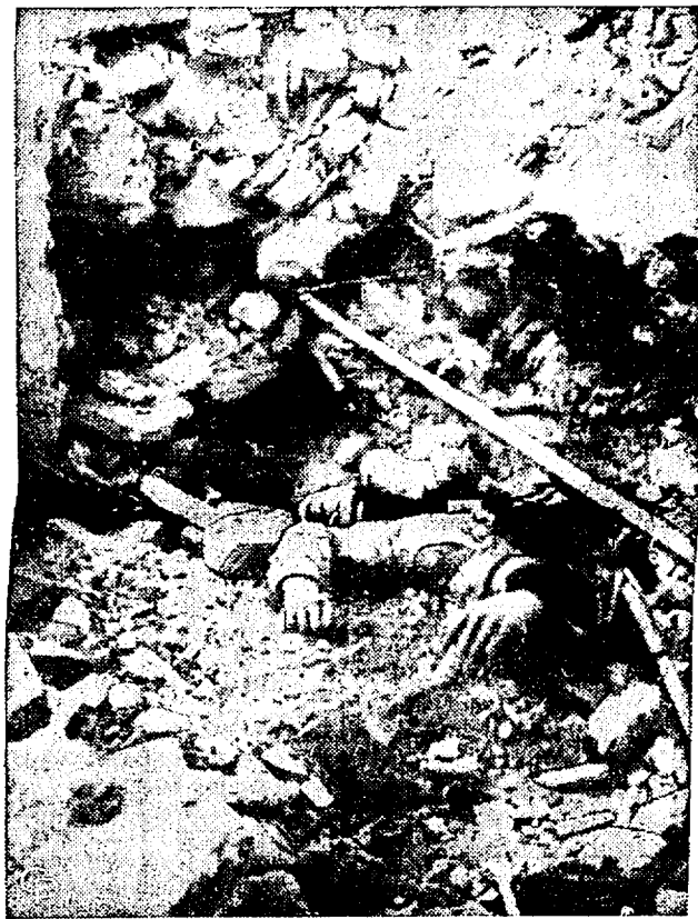
UNCOVERED BY AGADIR DEMOLITION CREW —Two of the uncounted thousands of victims of the earthquake, tidal wave and fire which leveled Agadir, Morocco, were uncovered by one of the demolition squads bulldozing and dynamiting the rubble. The once-proud port city is being leveled to avert epidemics. Authorities now estimate death toll at 10,000.
