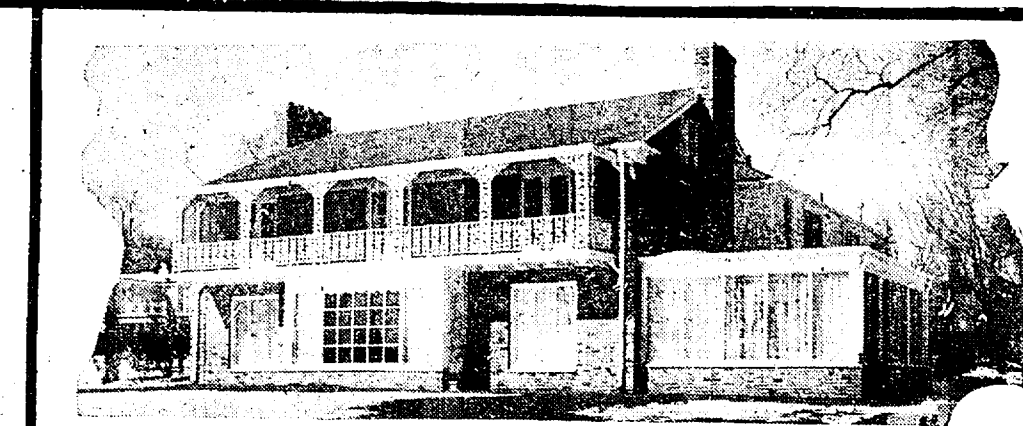
10 BEACON Architect, John L. Pottle
