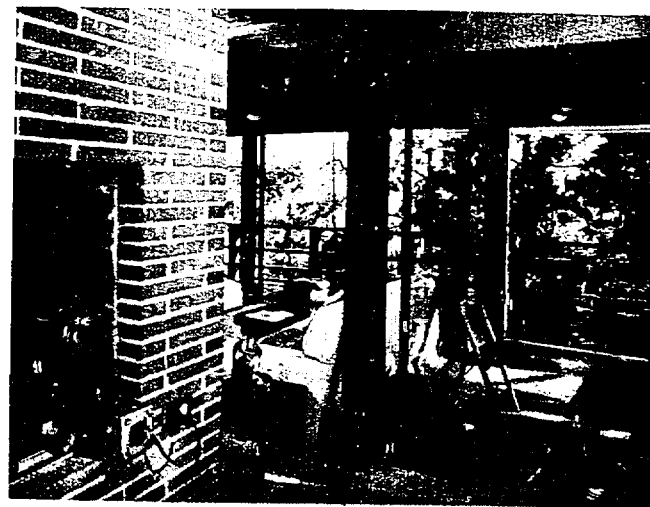
View of the living-room chimney, showing the space that is cut out on the kitchen side for an ample charcoal broiler.
