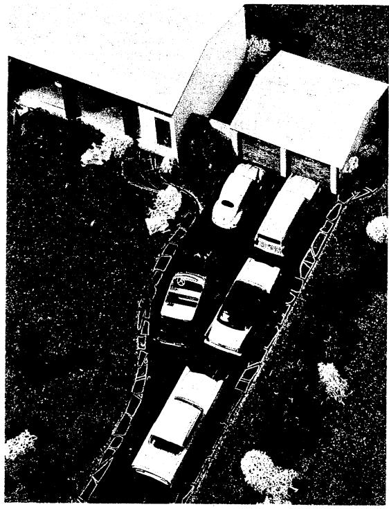
MODERN DRIVEWAYS are more than paved lanes from street to garage. If they are well designed, they offer an off-street guest-parking area with walk space between cars. Alighting passengers then use flanking "landing strips" as walks in order to pass cars and avoid wear and tear on lawn.
