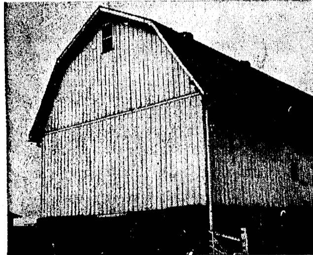
Shelter for livestock for protection against fallout was improvised in this barn by using bales of straw as a shield against potentially deadly "post-attack" radiation. Heavy concrete walls with straw shielding windows would protect livestock in pens on the barn's lower floor. Barn's upper floor (right) would be covered four bales deep directly above the pens. A shielded room for caretakers, and tractor-powered feed grinder and automatic feeder complete the shelter. OCDM Photo
