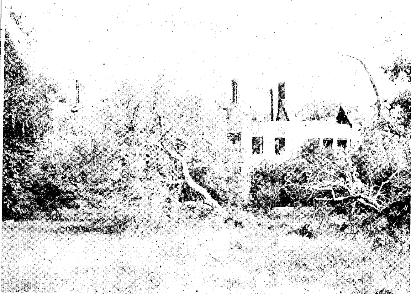
The former residence of the late Dr. and Mrs. Fred J. Murphy on the lakefront opposite Roosevelt place, was the scene of one of the Pointe's most spectacular blazes on Monday night. This was all that was left of the once-proud mansion on Tuesday morning.
