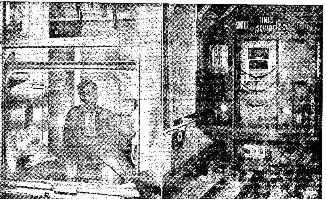
ROBOT TRAIN —Motorman Joseph A. Elender takes it easy in the New York Transit Authority's new "crewless" subway train, automated for the Grand Central-Times Square crosstown shuttle. Note the empty motorman's cab (left, photo right) as it pulls into Times Square. There will be a motorman and technician aboard for six months—testing.
