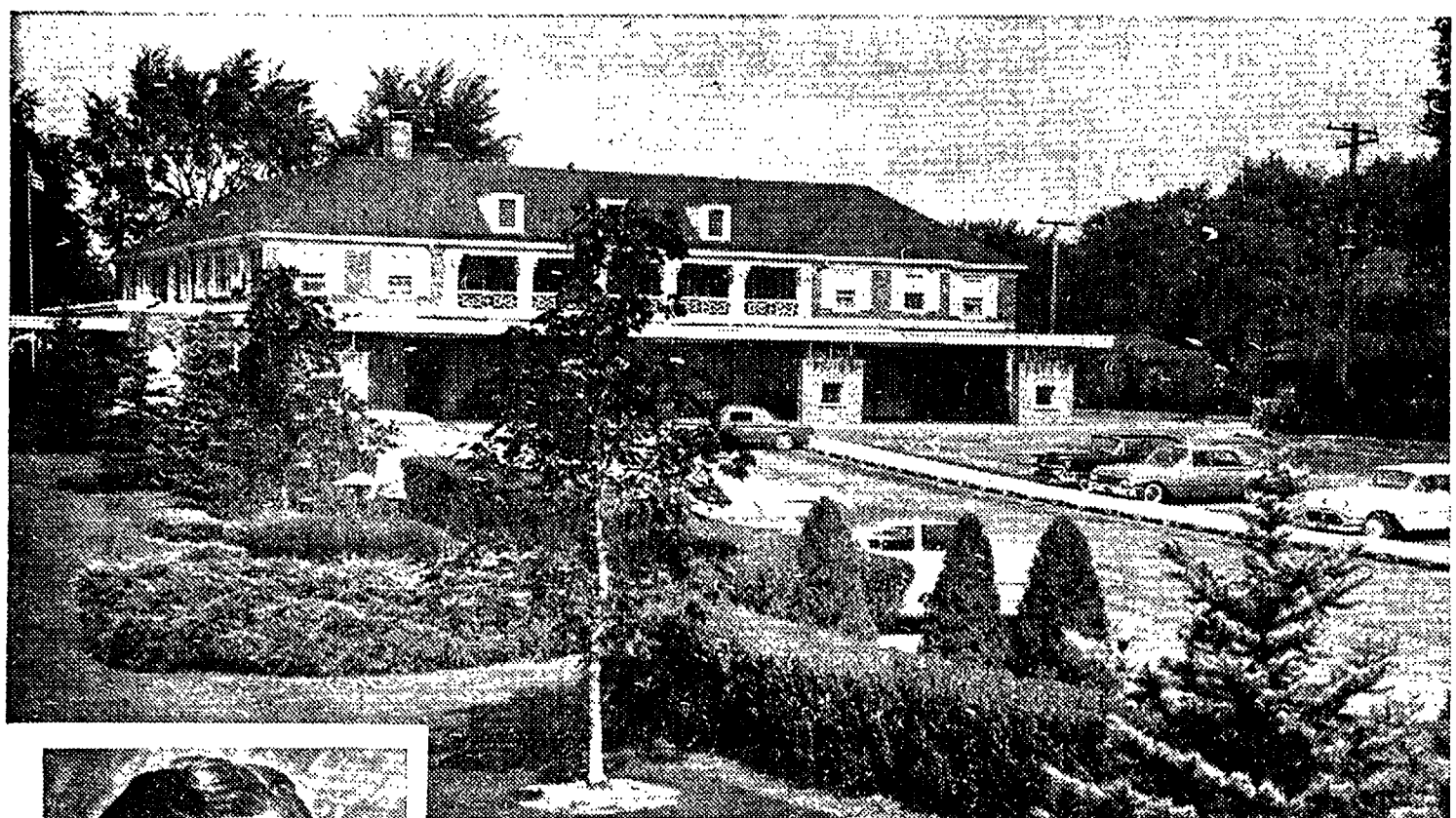
Rear of the Chas. Verheyden Funeral Home Showing Hidden Parking Area
