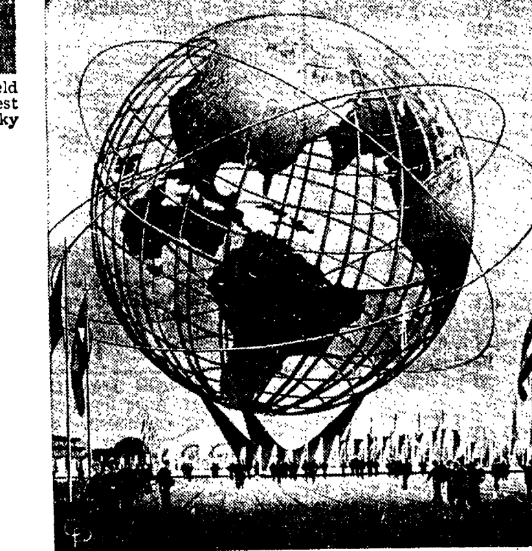
UNISPHERE —This sketch shows U.S. Steel's 12-story-high Unisphere, now under construction at the New York World's Fair site. It is of stainless steel, and designed to emphasize effect of lights playing on it. (Central Press)
