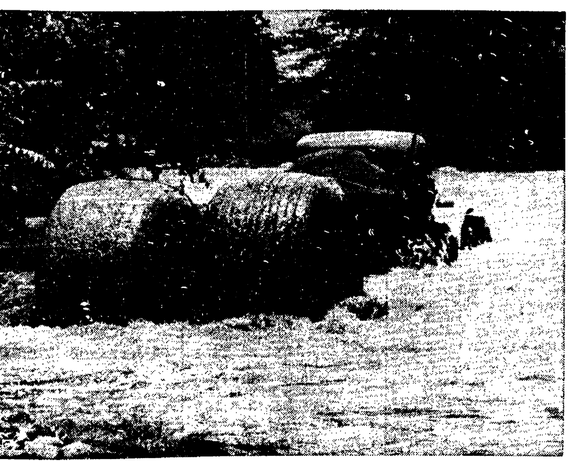
DAMP, THAT PAN-AM HIGHWAY —Tire-like Roll-Tankers sash through the residue of Panama's 300-inches-a-year rainfall as work progresses on the last 500 miles of the Pan-American Highway. This is jungle wasteland, and it took eight years just to survey the route. The highway building probably will run another eight, and cost maybe $100 million. The crews transport their fuel in these 500-gallon Roll-Tankers.
